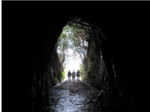
Stock tunnel, Marakopa
